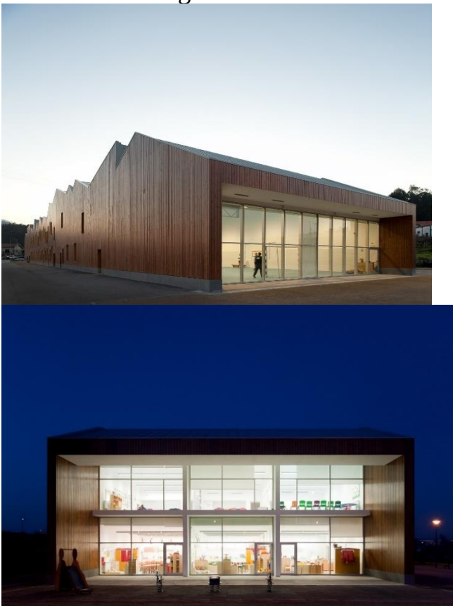
Figure 2 - 3 The glazed facades of the Mouriz School
