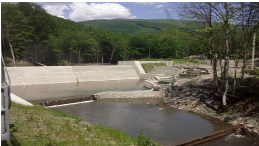
Water intake with a fish chute for the Shipit-2 mini-hydroelectric power station on the Turya River in the Transcarpathian region.
