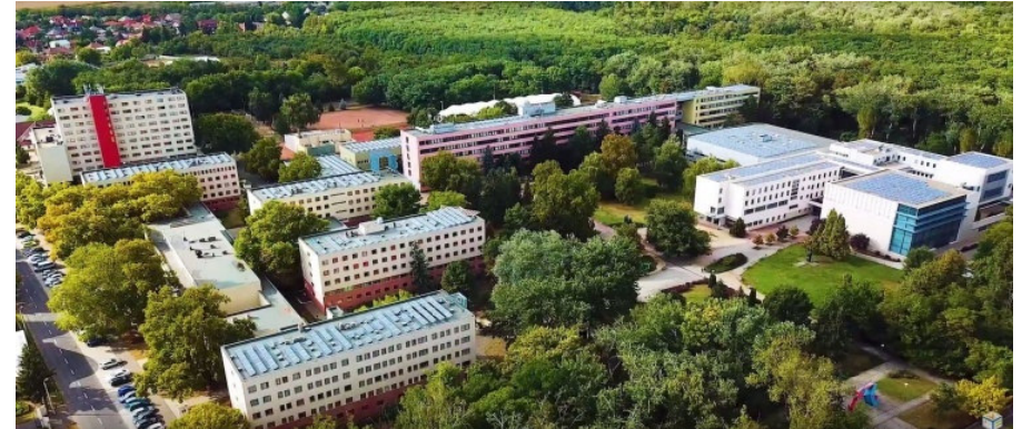
Aerial view of the campus, showing the PV panels installed on the roof of most buildings
