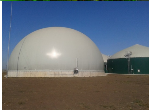
Biogas cogeneration power plant. Moara Commune, Suceava County
