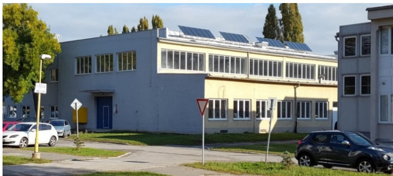
Fig. 1: Research center – solar collectors on the roof of the laboratory
