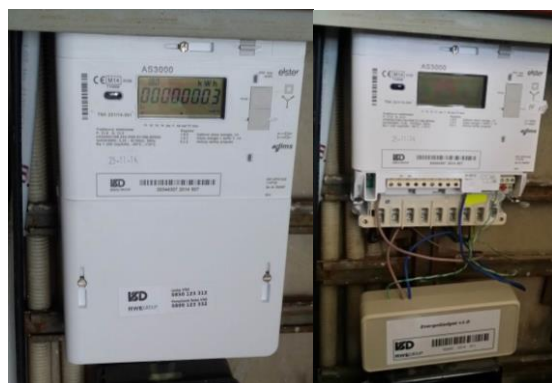
Figure 11. Mounting of the communication module
