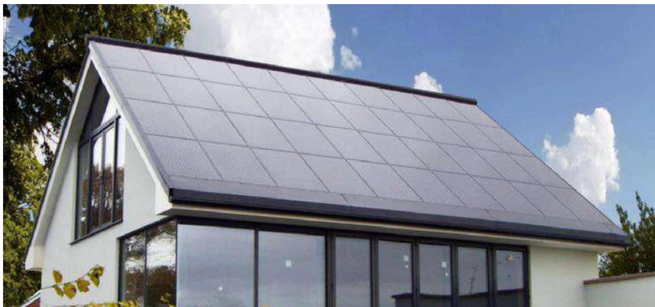
Рис.2.1. BIPV-модулі (Building-Integrated Photovoltaics)
